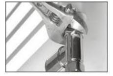
4. Insert the pipe (at this point you will have already prepared the water supply pipes to match up with the radiator or towel rail and valve dimensions). Then tighten the nut (with the olive already in place) that holds the pipe in position.
